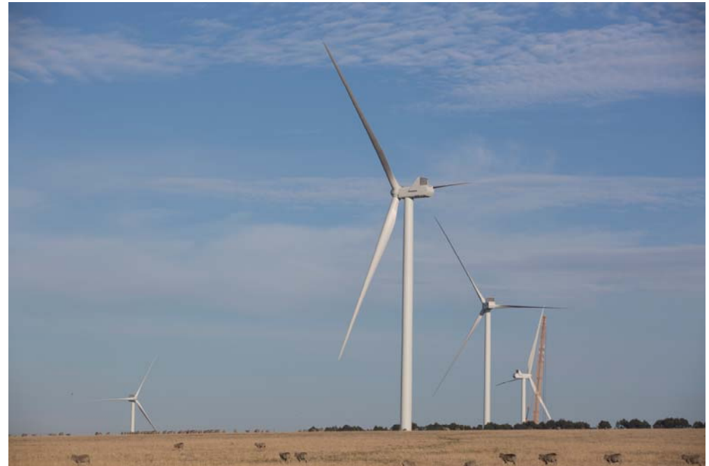
Salt Creek Wind Farm
