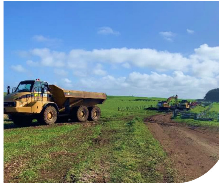
Civil works equipment onsite, establishing access
