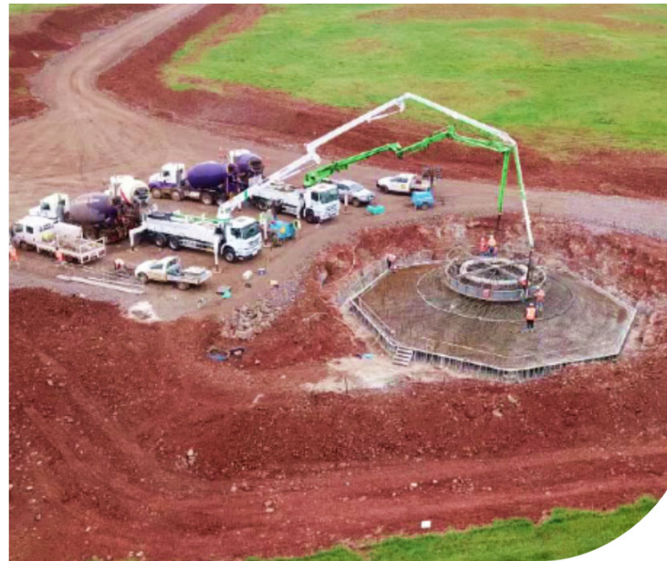
Wind turbine foundation being poured
