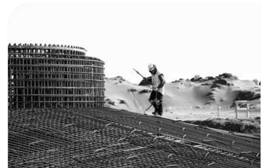
Above & right: Waipipi Wind Farm project team constructing wind turbine foundations.
