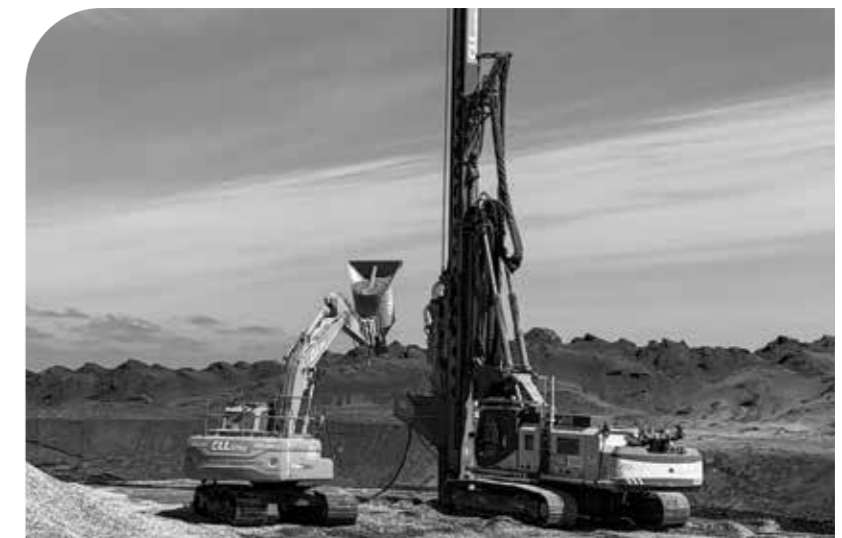
Left: Dynamic Compaction ground improvement works. Below: Rammed Aggregate Pier ground improvement works.
