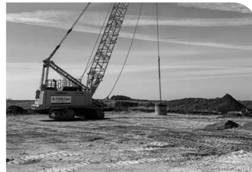
Left: Dynamic Compaction ground improvement works. Below: Rammed Aggregate Pier ground improvement works.
